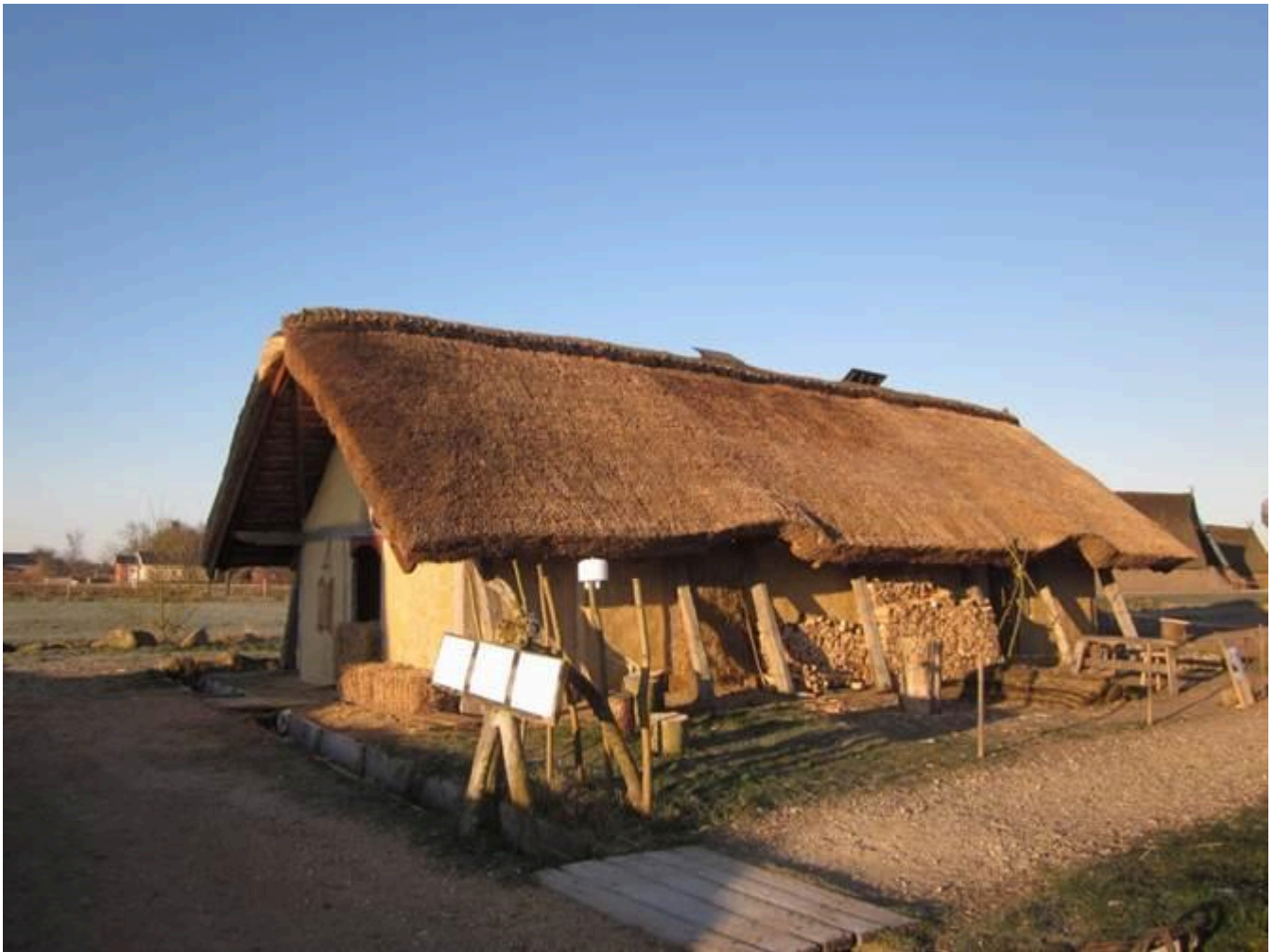
FIG 2. HOUSE 2 LOCATED AT BORK VIKING HARBOUR BUILT 2012.
