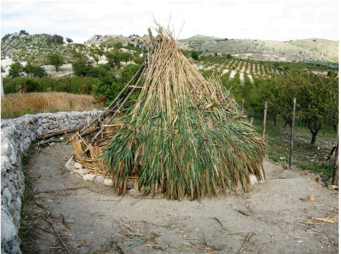
FIG 30. POSITIONING OF THE REEDS
