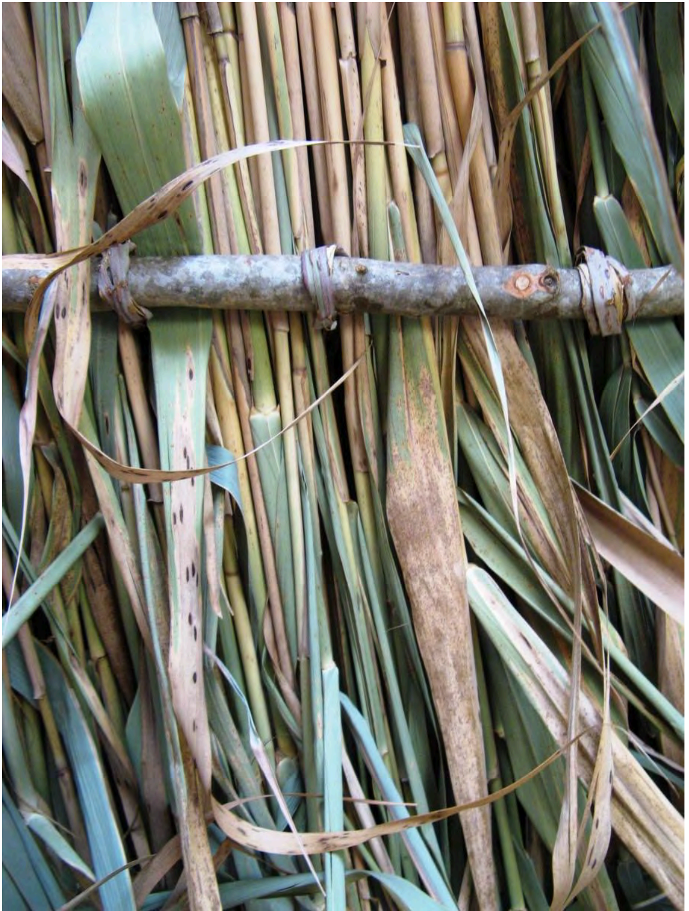
FIG 9. USE OF BLUEBERRY BRANCHES IN THE ROOF
