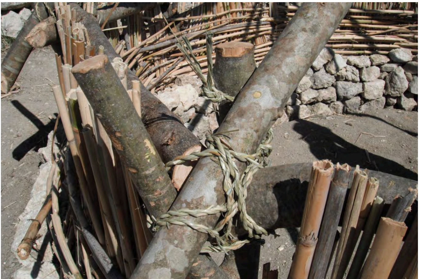
FIG 25. ROOF STRUCTURE - THE TIES
