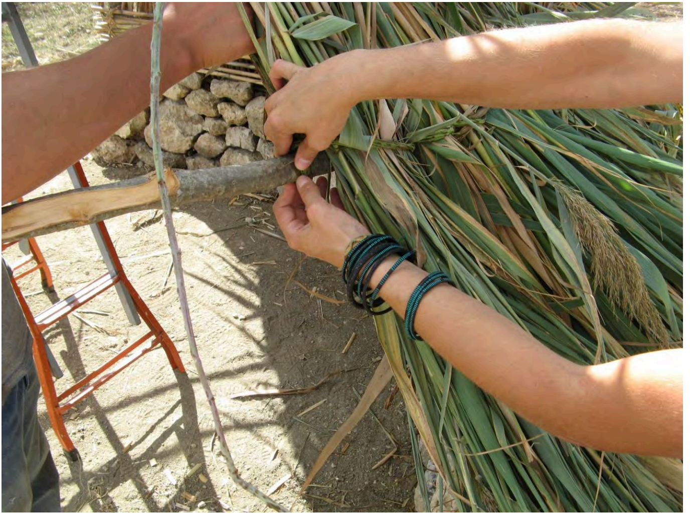
FIG 27. ROOF THATCHING - "SEWING" PROCESS
