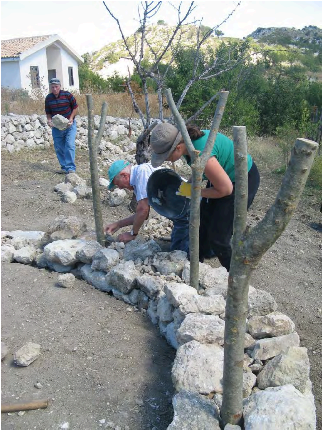
FIG 19. DRYSTONE WALL - BUILDING PROCESS
