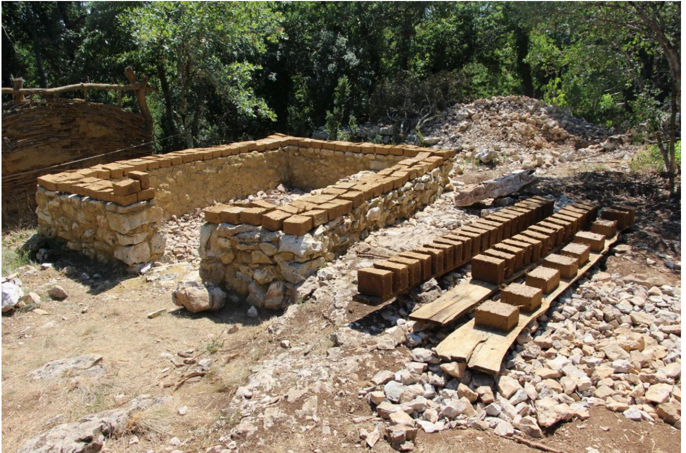
FIG 3. THE LIMESTONE FOUNDATIONS WITH THE FIRST OF ROWS OF ADOBE BRICKS. PHOTO BY RANDA ARDESCA
