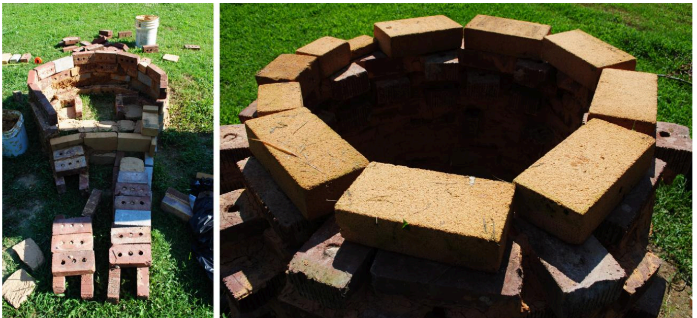
FIG 9. DEPICTIONS OF THE KILN ARE ABOVE AND REPRESENT NUMEROUS THINGS. (LEFT) SHOWS THE GRADUAL GROWTH THE KILN WOULD UNDERGO WHILE (RIGHT) IS TOWARDS THE END OF CONSTRUCTION. (RIGHT) IS THE APPLICATION OF FIREBRICKS LOCATED ON THE TOP OF THE KILN. THESE WERE ADDED TO ACT AS A BARRIER BETWEEN THE INDUSTRIAL BRICKS AND THE TEMPORARY DOME. THE GOAL HERE WAS TO ALLOW FOR THE DOME TO BE FIRED WHILE NOT STICKING TO THE KILN. PHOTO BY BRIANNA JENKINS
