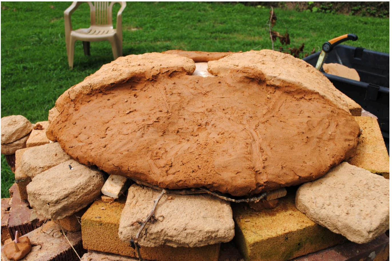
FIG 10A. DISPLAYS THE TEMPORARY DOME PROCESS. THERE WERE TEN MUDBRICKS MADE SPECIFICALLY FOR THE DOME, HOWEVER AFTER SUNBAKING ONLY TWO SURVIVED AND WERE USED. THE MEASUREMENTS WERE AS FOLLOWS: .406M LONG AND .254M AT THE LONGEST WIDTH. THOSE TWO WERE ADDED TOGETHER WITH COILS OF THE RED LOCAL CLAY. PHOTO BY BRIANNA JENKINS
