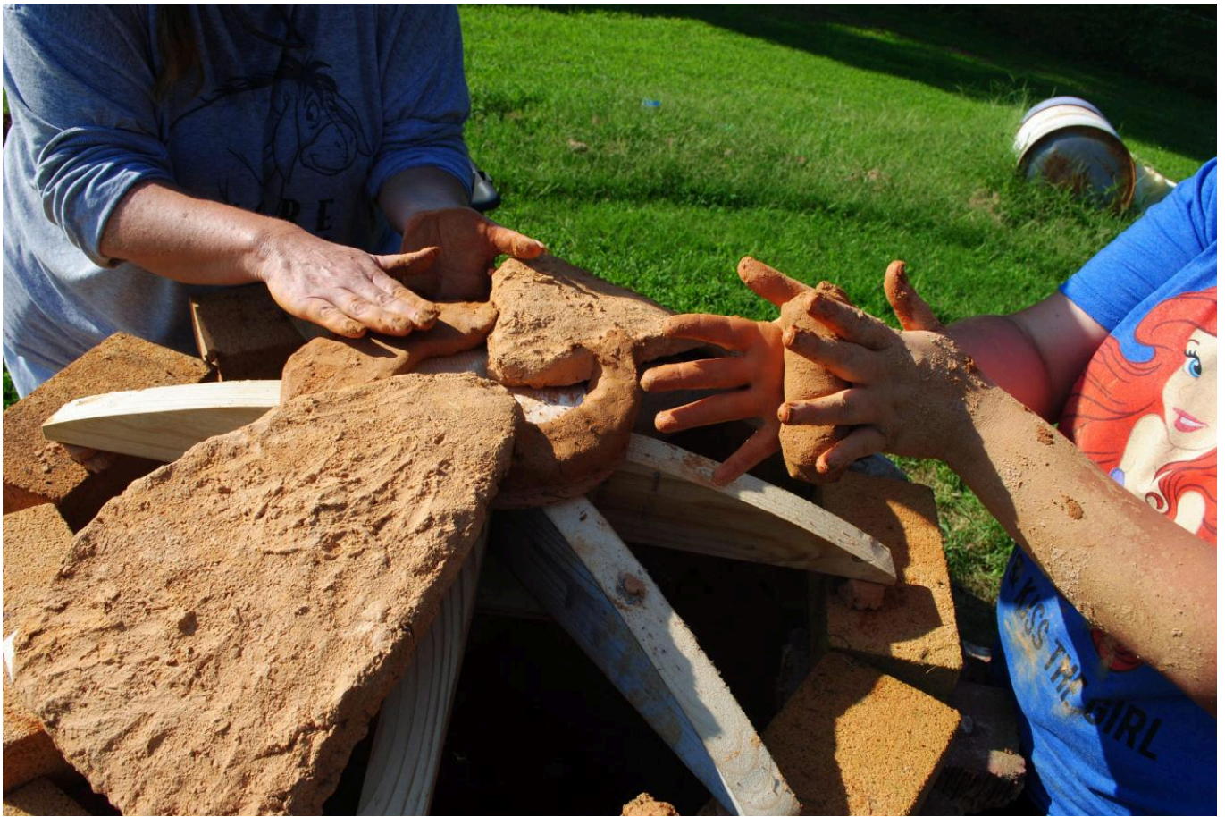
FIG 10A. DISPLAYS THE TEMPORARY DOME PROCESS. THERE WERE TEN MUDBRICKS MADE SPECIFICALLY FOR THE DOME, HOWEVER AFTER SUNBAKING ONLY TWO SURVIVED AND WERE USED. THE MEASUREMENTS WERE AS FOLLOWS: .406M LONG AND .254M AT THE LONGEST WIDTH. THOSE TWO WERE ADDED TOGETHER WITH COILS OF THE RED LOCAL CLAY. PHOTO BY BRIANNA JENKINS
