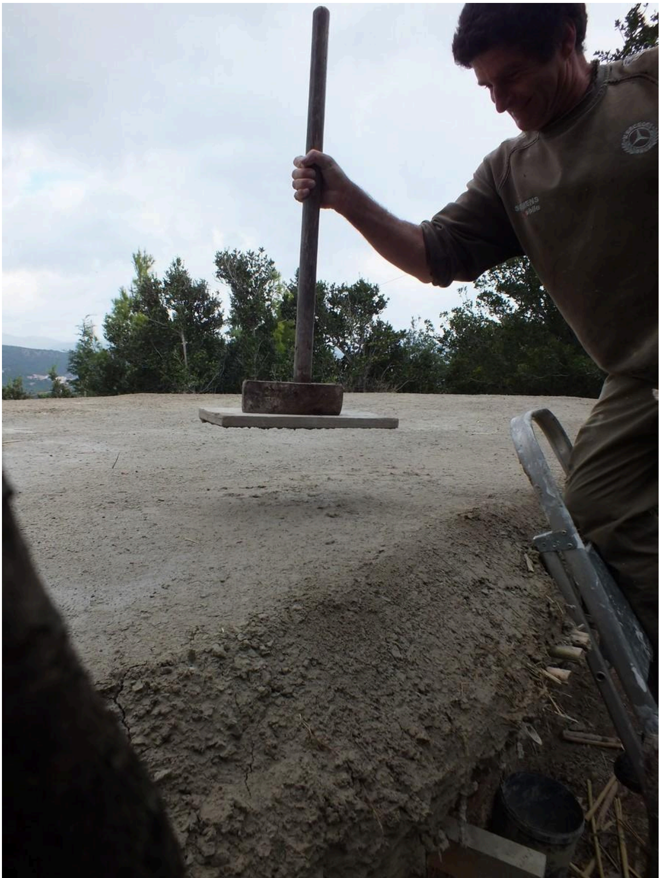
FIG 23. COMPRESSING THE LAST ROOF LAYER.
