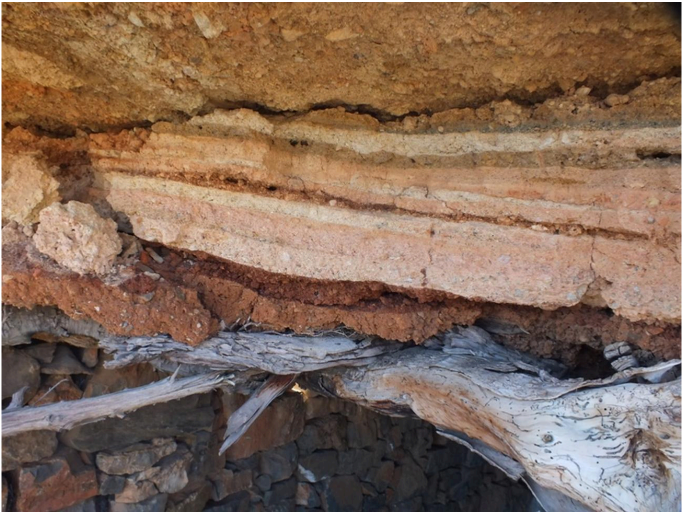
FIG 21. LAYERING IN A TRADITIONAL CRETAN ROOF (CURRENTLY CRUMBLING). ALL THE VISIBLE LAYERS WERE AT SOME POINT TOPPED WITH CEMENT WHICH PRESERVED THE STRATIGRAPHY USUALLY LOST.
