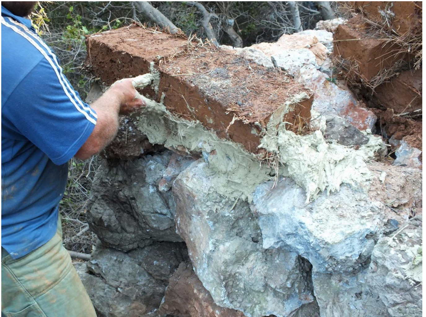
FIG 13. THE FIRST LAYER OF TWO DAY OLD MUDBRICKS, USING KOUSKOURAS-BASED MORTAR MIXED WITH FINER STRAW.
