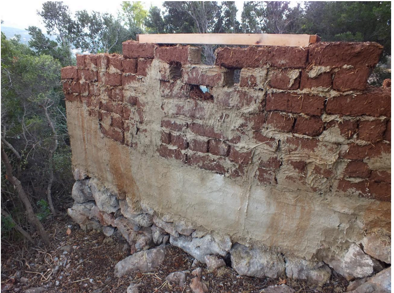
FIG 8. THE SOUTHERN WALL WITH THE "WINDOW" DURING THE FIRST RAIN, BRICKS BROWN, MORTAR AND PLASTER BEIGE, THE SLIGHT AMOUNT OF BRICK DISSOLVED BY RAIN IS VISIBLE AS DARKER STAINS ON THE BEIGE SURFACE (PRODUCED DURING CLOSING PERPENDS). THE FOUNDATION STONES ARE NOT FILLED IN.
