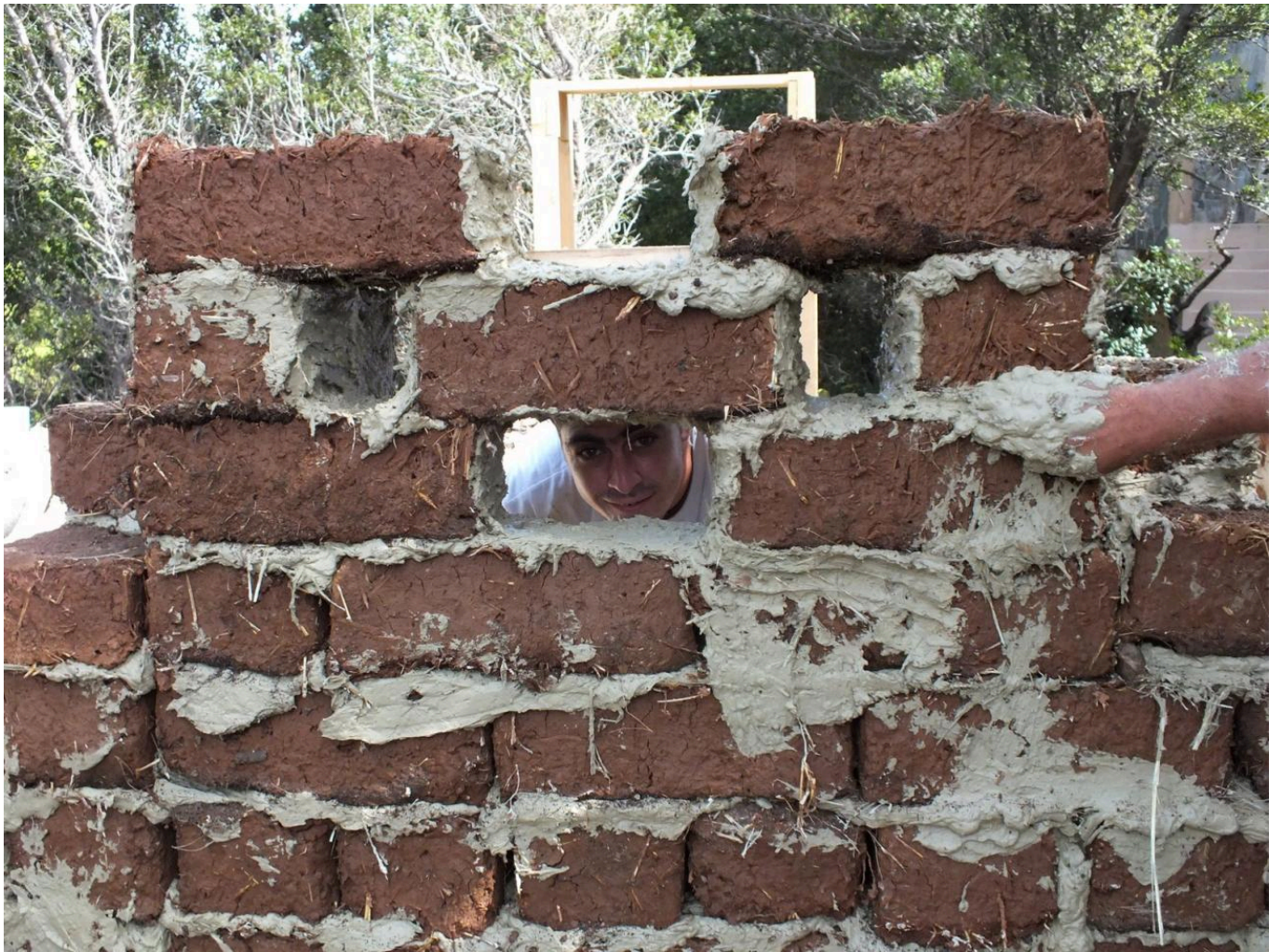
FIG 16. MINOAN STYLE "WINDOW" CREATED BY SPACING A SINGLE ROW OF BRICKS.
