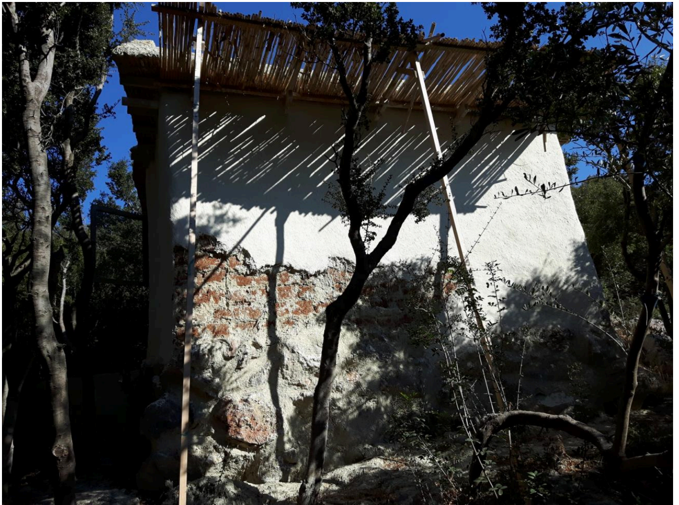
FIG 26. THE WEATHER SIDE WALL SINCE THE DAMAGE IN JANUARY 2015 WITH THE GIANT CANE RAFTERS PROTECTING THE WALL FROM FURTHER HARM.
