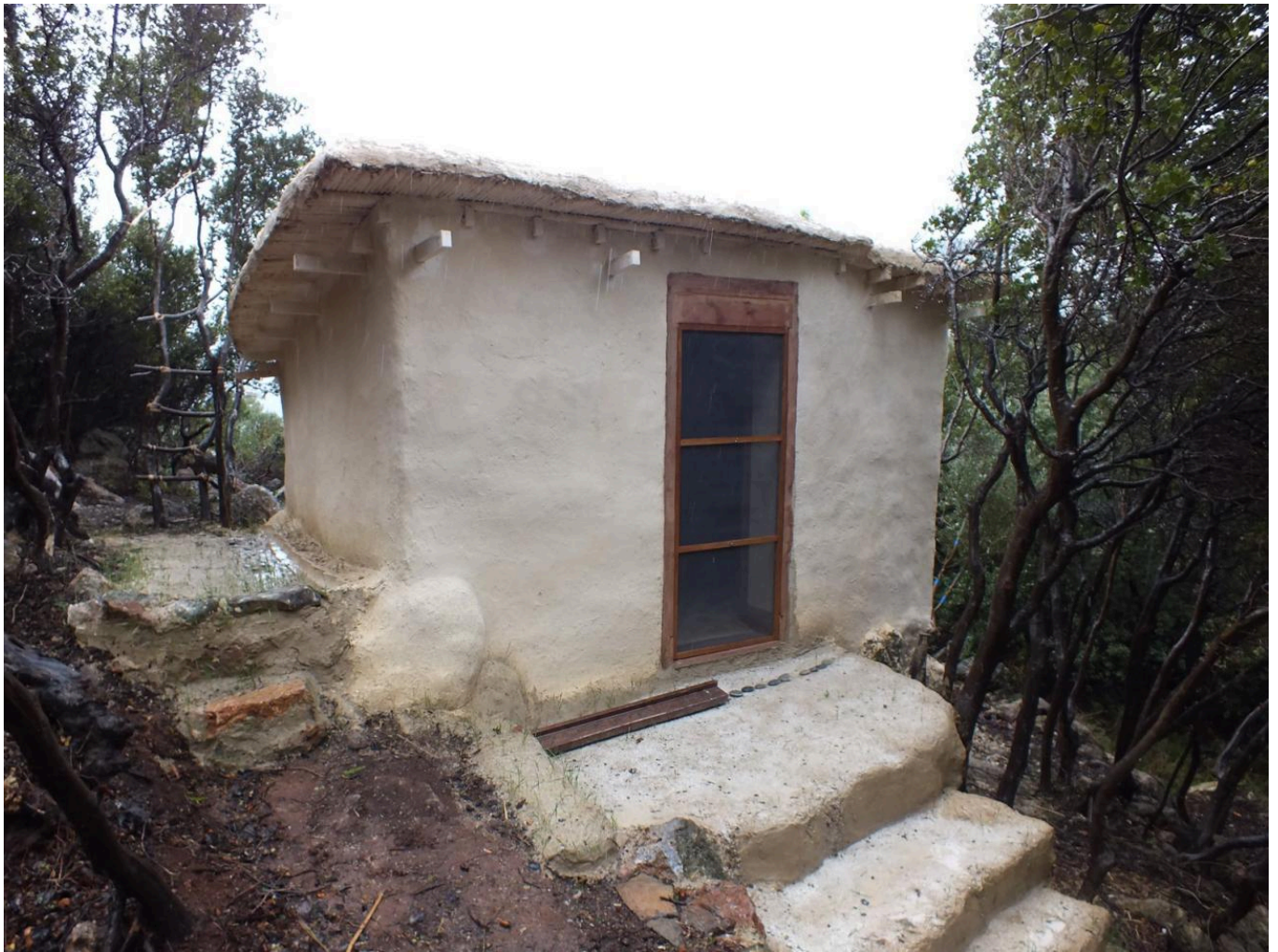
FIG 27. THE EXPERIMENTAL HOUSE JUST FINISHED WITH ITS TREE LADDER TO GET ON THE ROOF, THE DRAIN, THE PEBBLES UNDER THE DRIPPING RAFTERS AND THE PRELIMINARY DOOR, 12/2014. ON VARIOUS SURFACES CEREALS CAN BE SEEN SPROUTING FROM THE CLAY-CHAFF MIXTURE.
