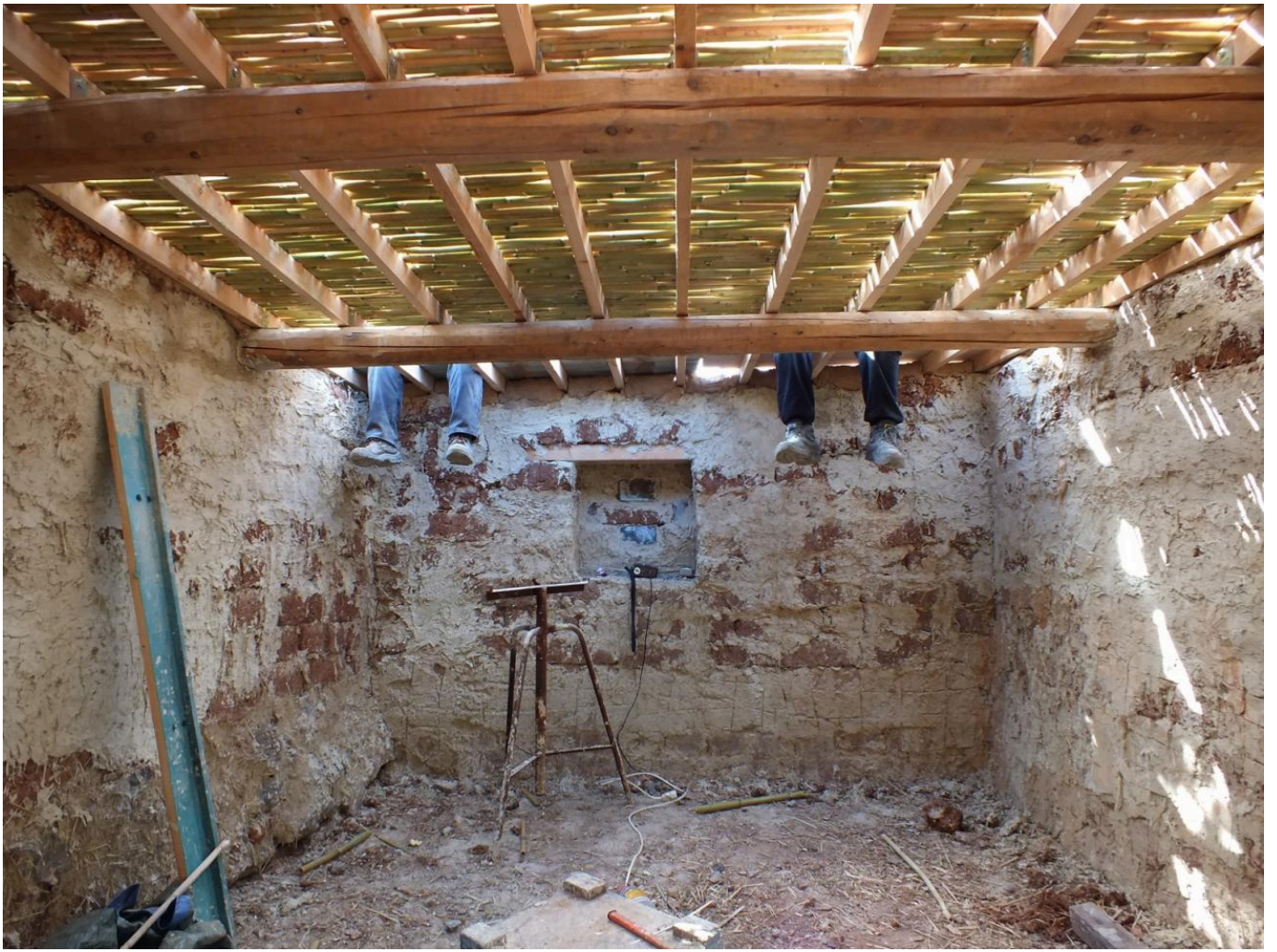
FIG 22. THIN BEAMS AND GIANT CANE AS FIRST ROOF LAYERS OVER THE MAIN BEAMS.
