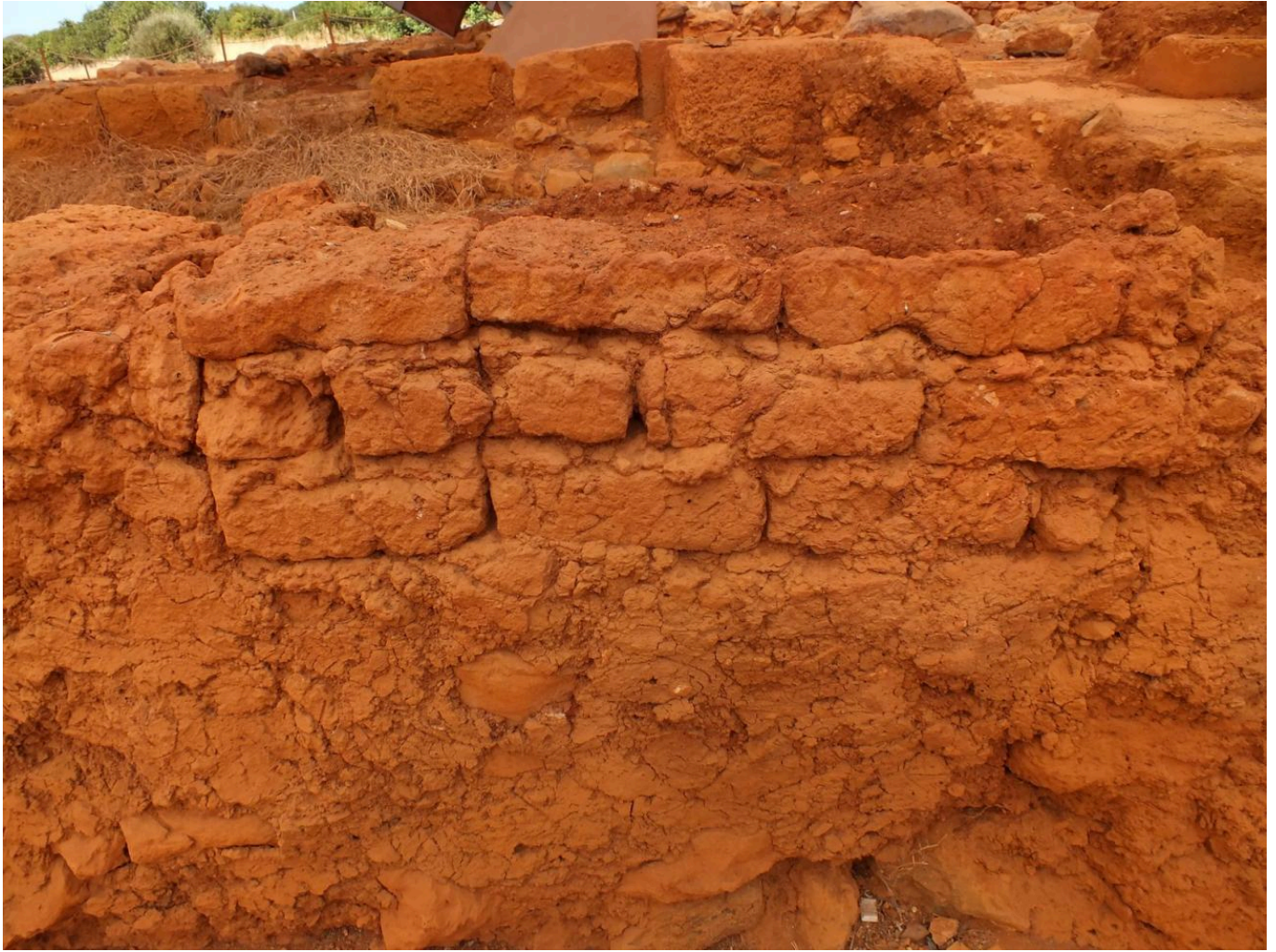
FIG 6. MALIA QUARTIER MU MUDBRICK WALL WITH SEVERAL PERPENDS ALIGNED.
