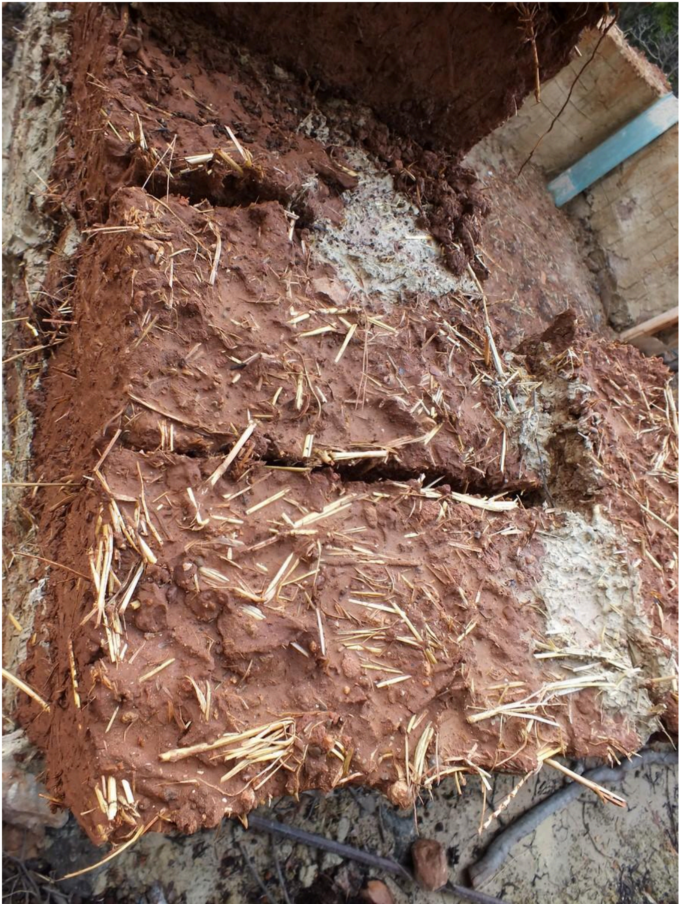
FIG 18. BUILT MUDBRICKS AFTER THE FIRST STRONG RAIN. THE SURFACE SHOWS ONLY SOME CLEAN-WASHED STRAW HAULMS.
