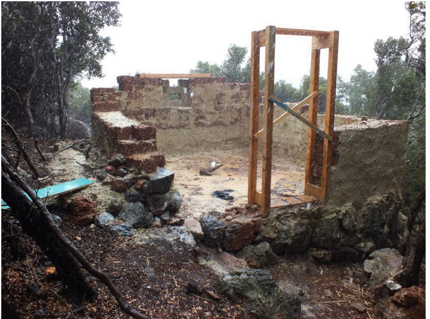
FIG 17. RAISING THE MUDBRICK WALLS -HEADER AND STRETCHER ALTERNATING- BUT NOT BY LAYER. THIS FIRST RAIN CAME EARLY IN 2014.
