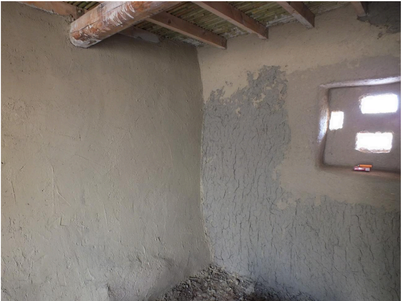
FIG 24. ROUGHCAST AND FINAL RENDERING OF THE PLASTER.
