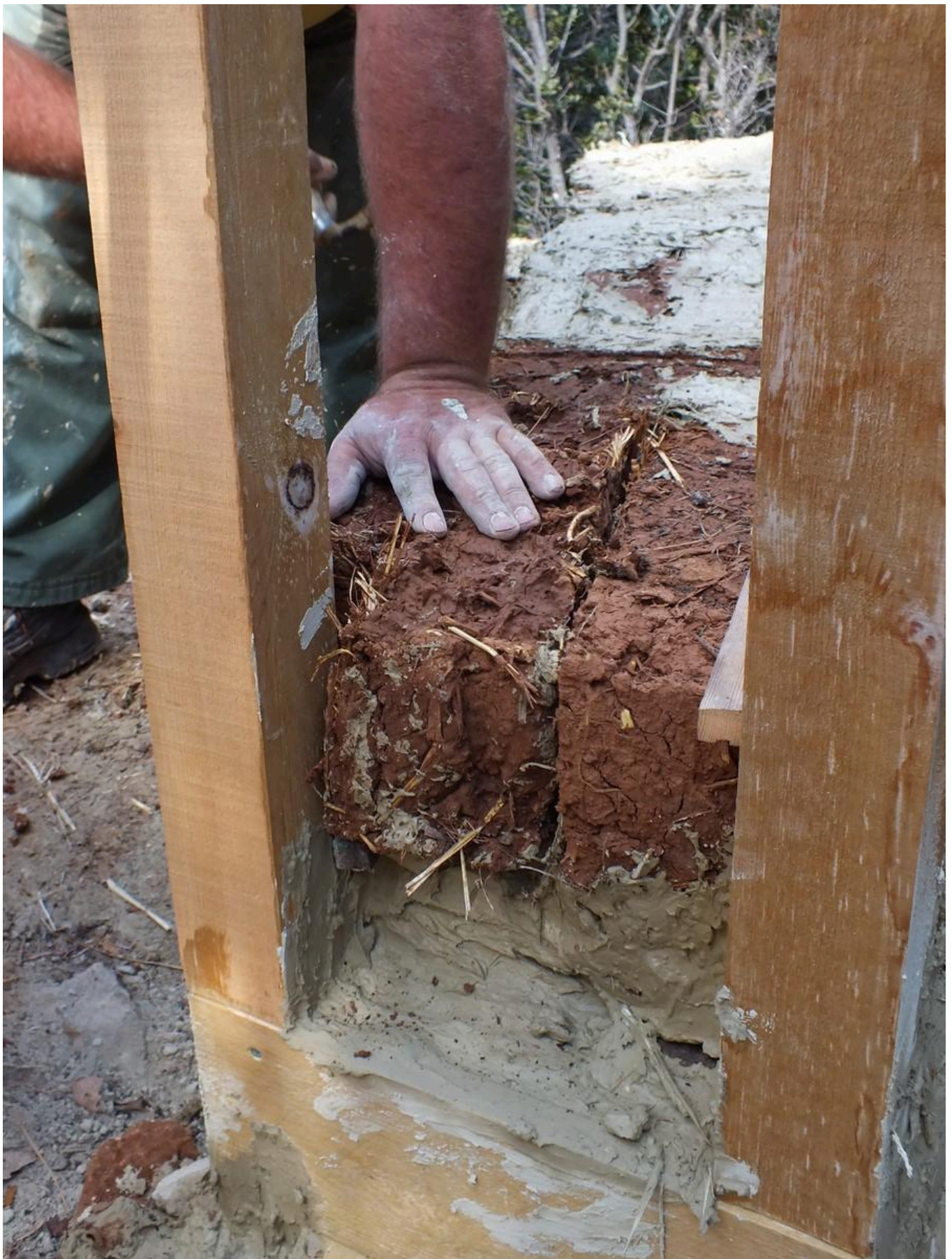
FIG 15. MUDBRICKS WITH CUT EDGES TO PROVIDE A BETTER BONDING WITH THE DOOR CASING.
