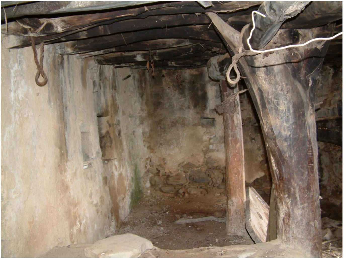
FIG 20. TRADITIONAL CRETAN ROOF CONSTRUCTION - THE TIMBER IS HERE PROBABLY OAK (SOOT-BLACKENED).THE WALLS ARE RUBBLE BUILT WITH MUD MORTAR, MUD PLASTER AND LIME PAINT.
