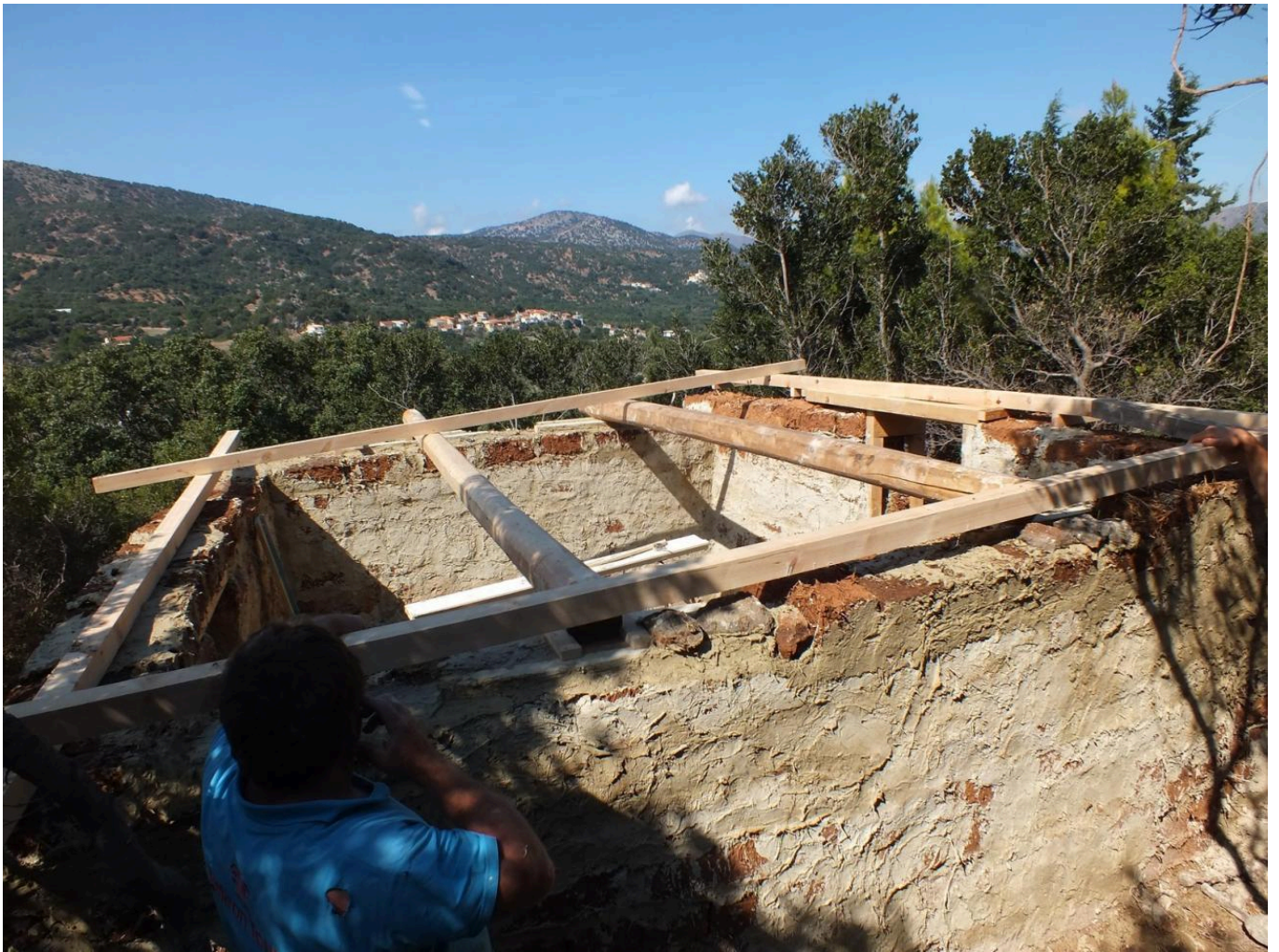
FIG 19. THE BASIC ROOF CONSTRUCTION - BEAMS BEDDED IN COB WITH A RINGBEAM ON TOP. THE SPACES UNDERNEATH ARE LATER FILLED WITH COB.
