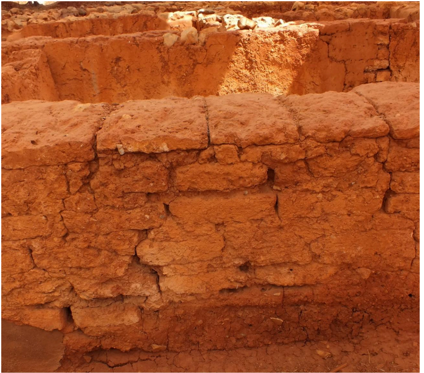
FIG 7. MALIA QUARTIER MU MUDBRICK WALL WITH OFFSET PERPENDS.
