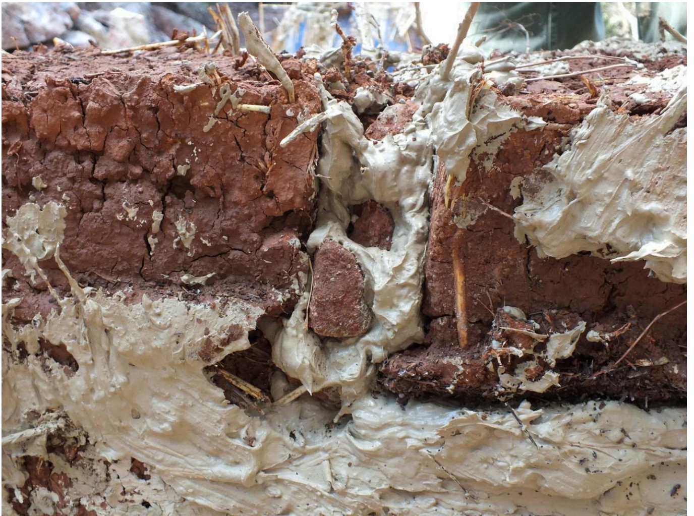
FIG 14. MUDBRICK WALL WITH KOUSKOURAS MORTAR USING ADDITIONAL STONES TO FILL GAPS.
