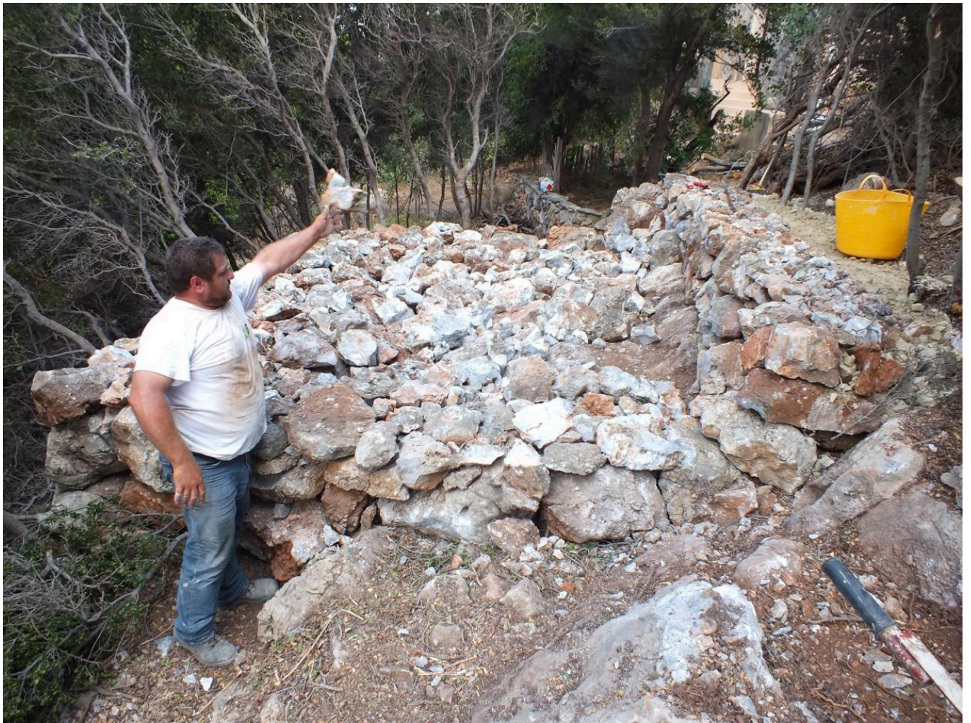
FIG 10. FILLING THE ONCOLITHIC FOUNDATION WITH RUBBLE AND THE UPSLOPE SIDE WITH WATERPROOFING CLAY OVER RUBBLE.
