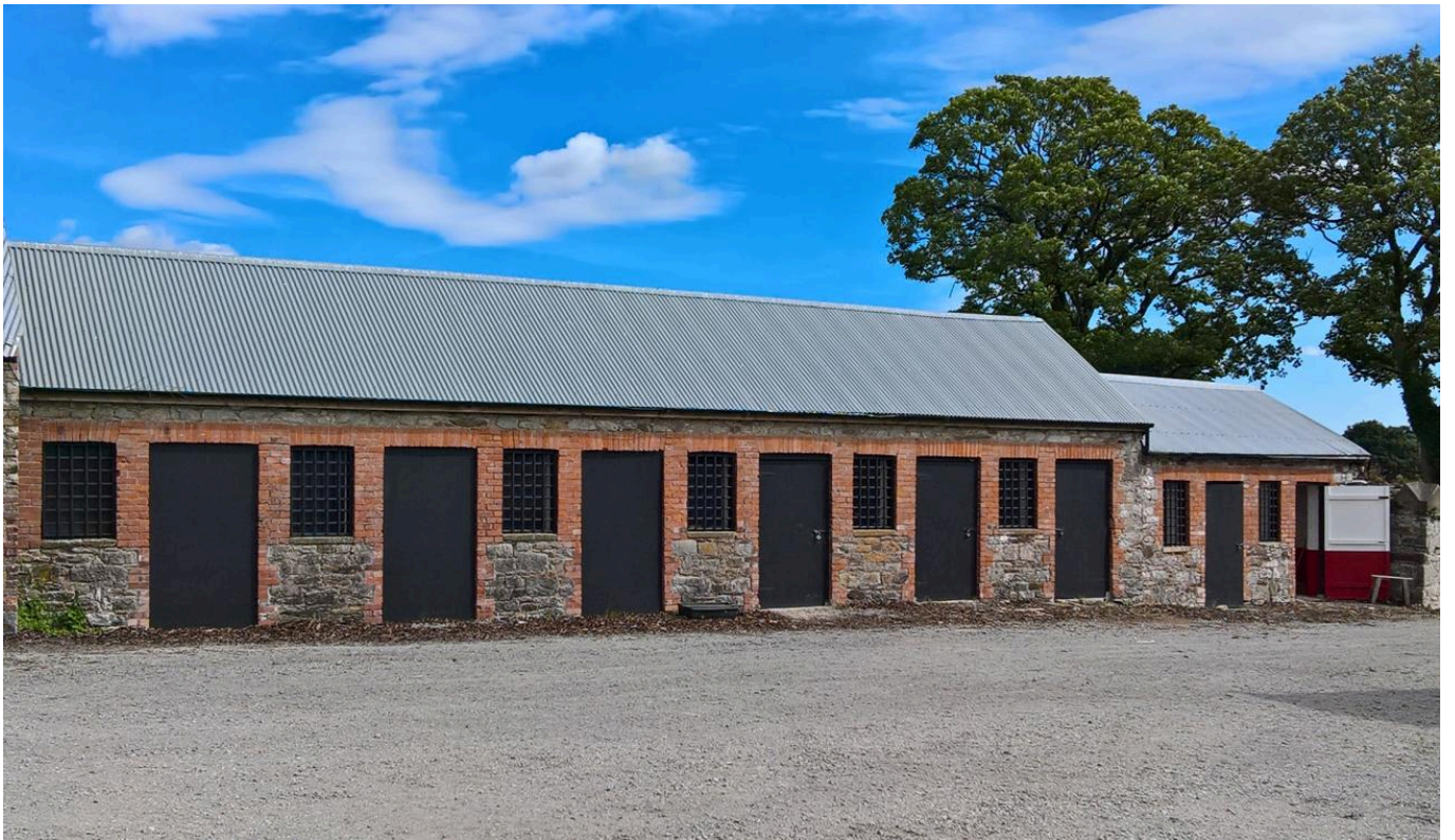
FIG 3. FIRST PHASE OF CONVERSION COMPLETE
