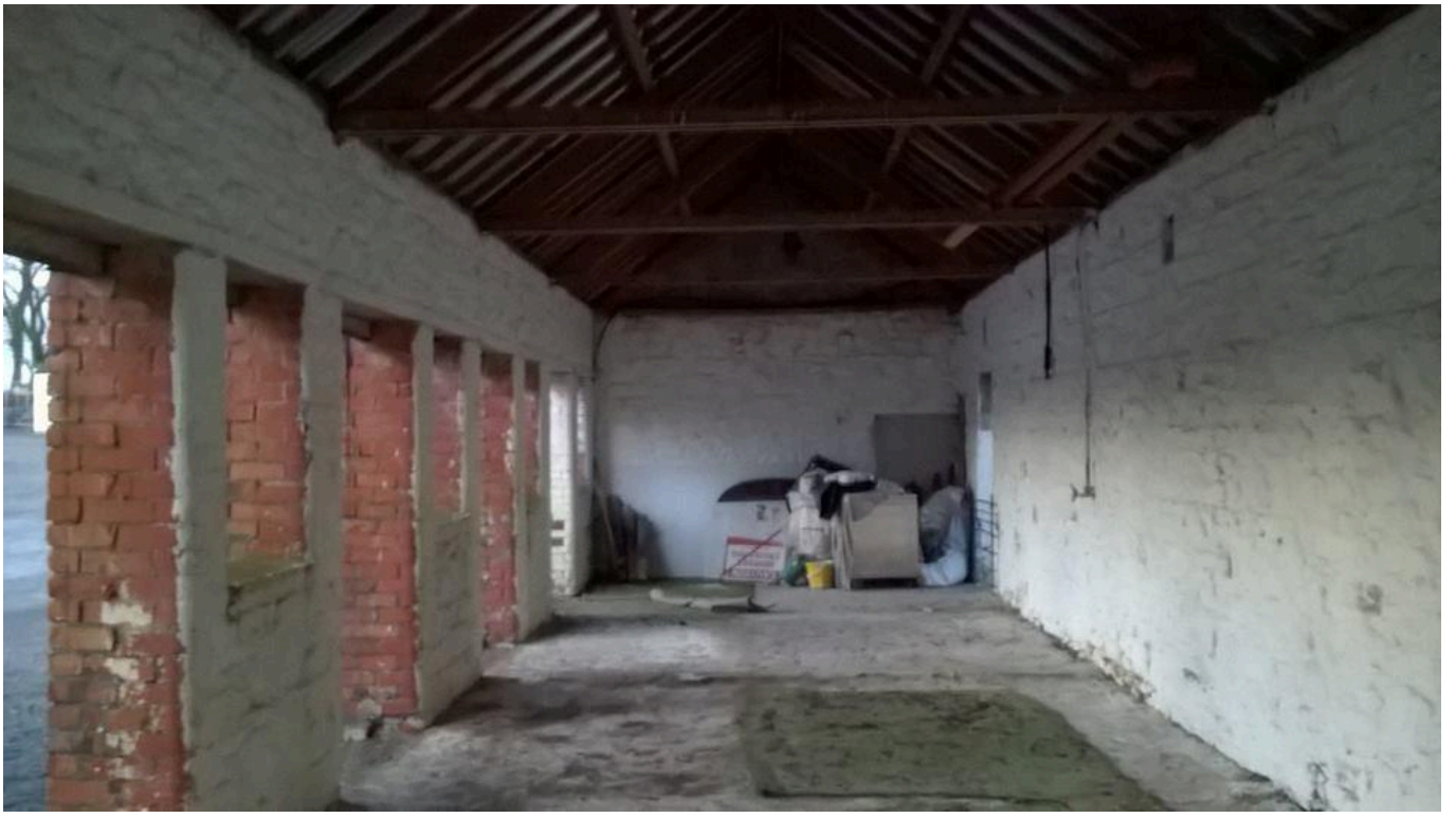
FIG 2. BUILDING INTERIOR IN 2015
