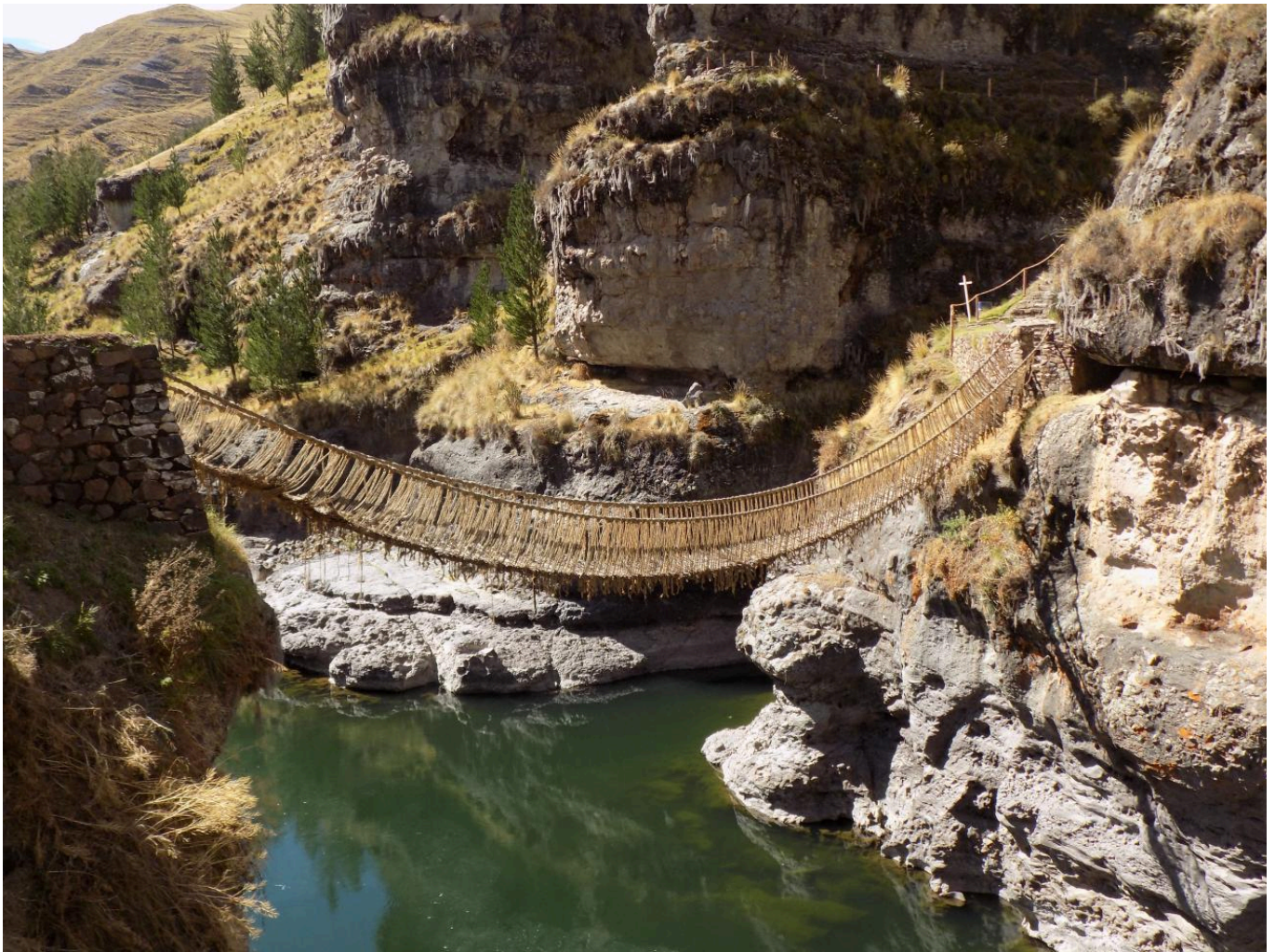
FIG 4. THE Q'ESWACHAKA BRIDGE IN PERU, HAND WOVEN ANNUALLY BY THE NEIGHBORING VILLAGERS. COPYRIGHT: MAUREEN FOLK (US)
