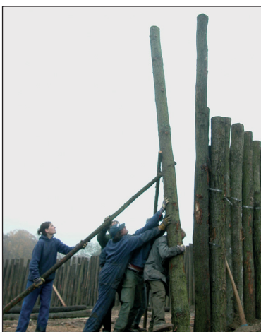
■ Fig. 4 The posts of the palisade were erected by hand.
