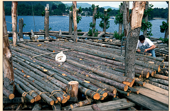
■ Fig 3. Alder floor timbers of the reconstruction based on original floor from Oakbank Crannog.
