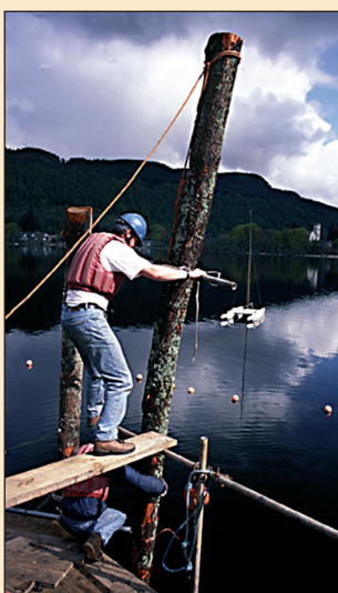
■ Fig. 4 Driving piles at the reconstruction.
